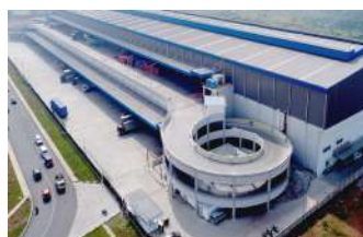
West Cikarang Warehouse, Bekasi
